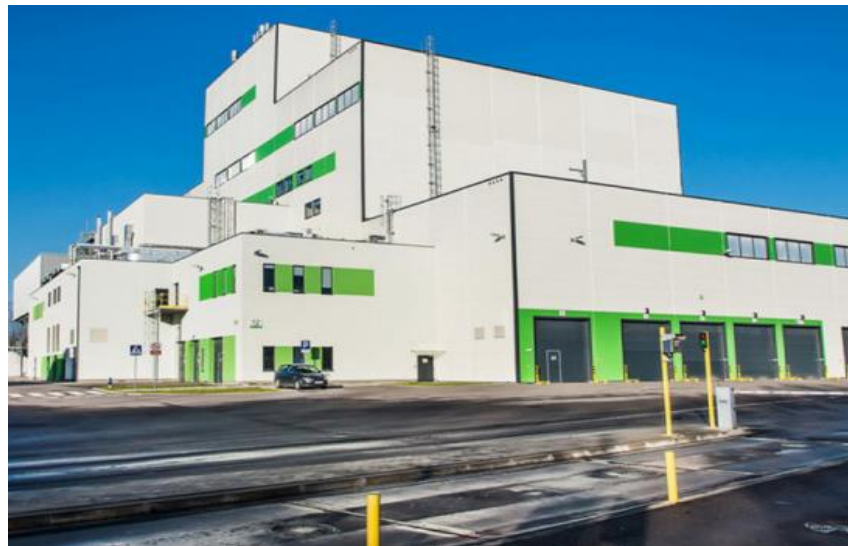
NID - Novel Intergrated Desulphurisation
